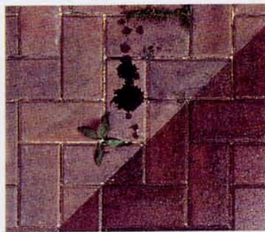
Figure 2: Contrast between untreated blockwork and blockwork treated with a polyurethane-based preparation.
