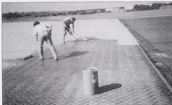
Figure 3. Applying Polymer Stabilisers
