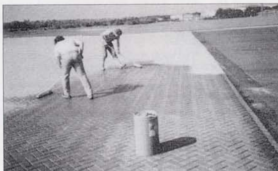
Figure 3. Applying Polymer Stabilisers
