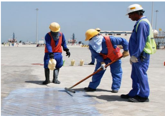
Application via gauging pot and application squeegee.
