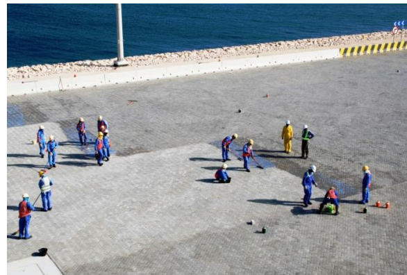
Application in controlled bands of 10 meters.
